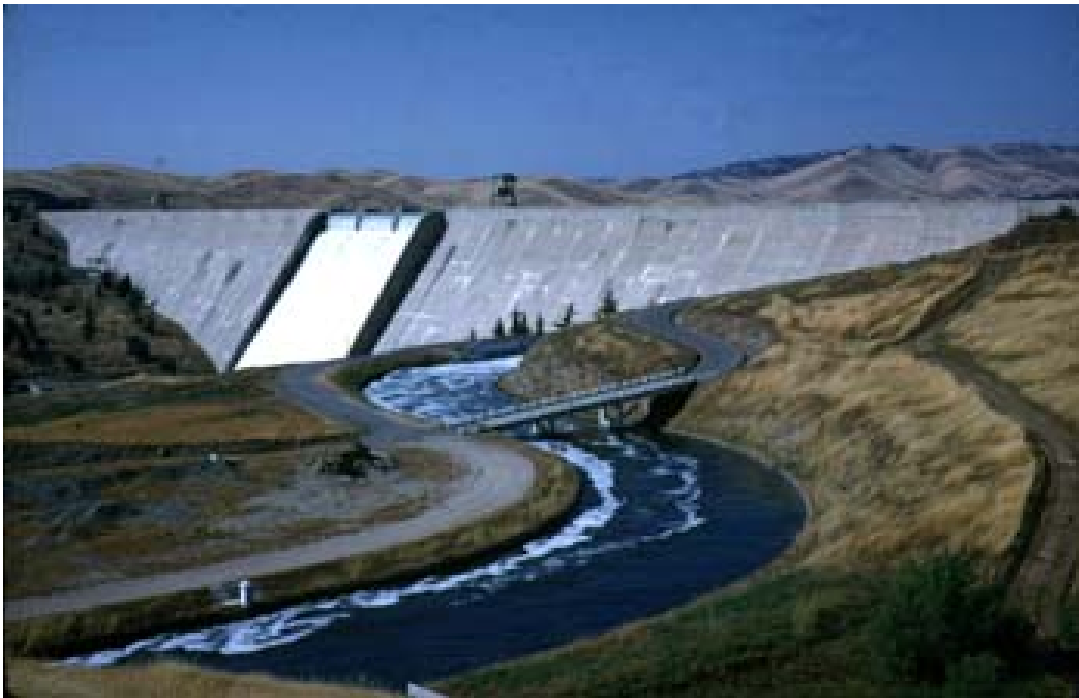
Figure 2 - Friant Dam downstream face.
